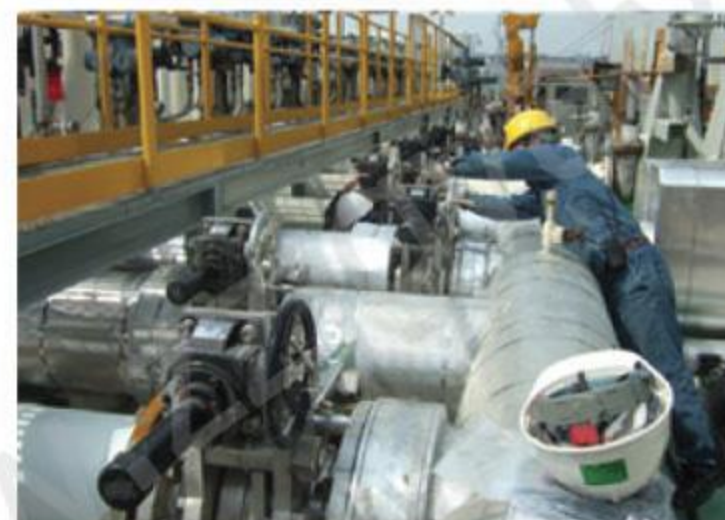
Loading Arm Construction
